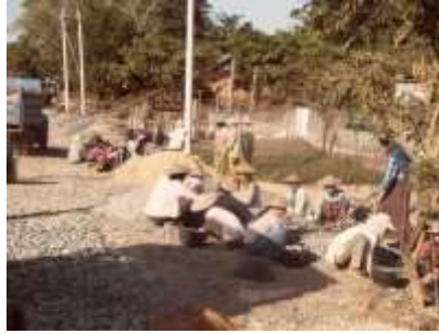
Figure 2: Road under Repair
